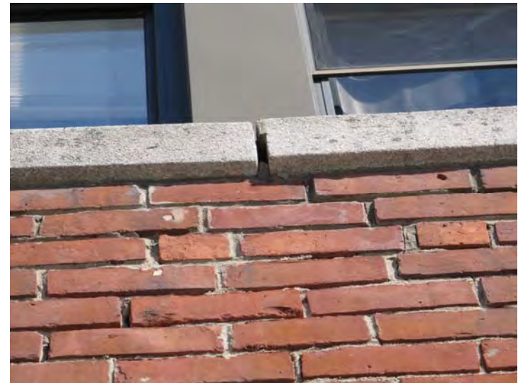
Mortar loss between sections of windowsill is widespread
