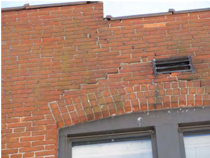
Cracks/mortar loss evident at various locations in masonry exterior wall surfaces
