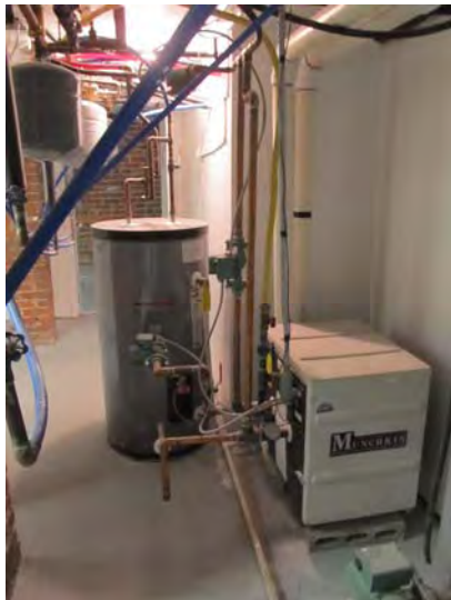
One of two recently installed boilers and indirect-fired domestic hot water tanks – No problems related to equipment observed or reported
