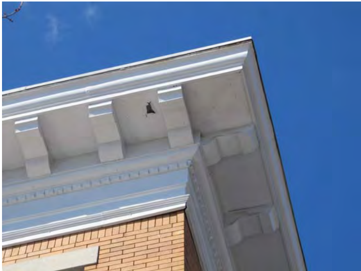
Metal cornicing is in need of surface preparation and painting
