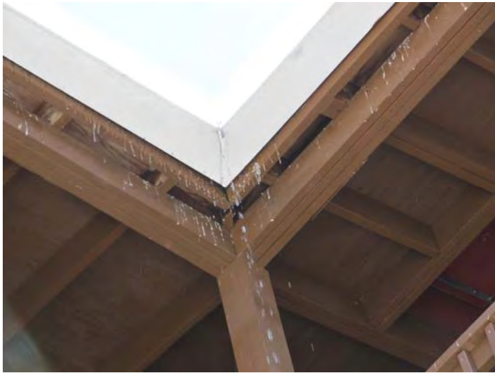
Gutter at stair/deck structure is leaking at the inside corner and needs replacement
