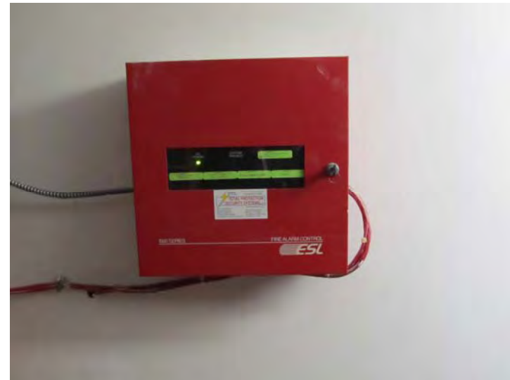
Original zone-type fire alarm control panel is serviceable but at or near the end of its expected useful life
